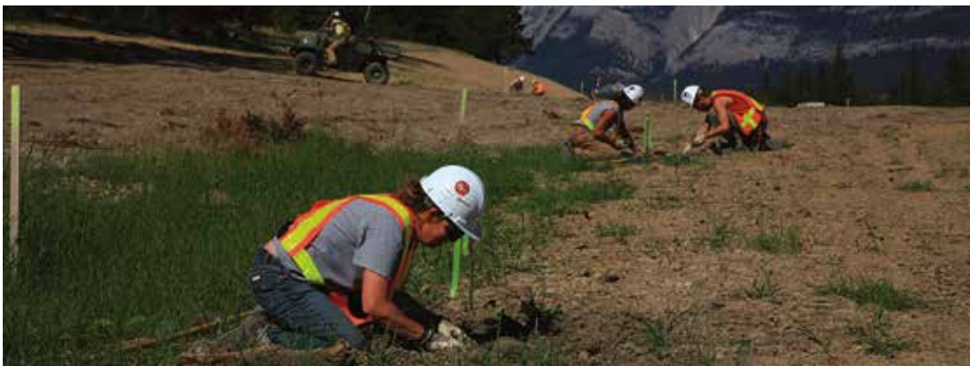
Surveying the right-of-way in advance of construction.
